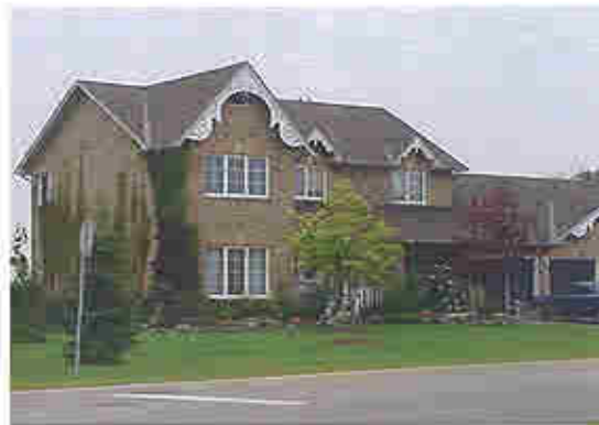
Cranston Drive -- This new home represents an appropriate adaptation of the historical precedents, with buff brick, cross-gables, decorative masonry over the windows, and decorative verge boards.
