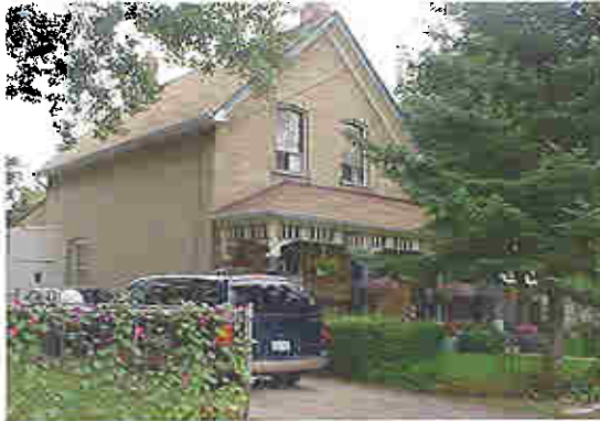
Cedar Street -- This Queen Anne, front-end gabled house has a decorative, full-length spindlework porch. The slightly curved windows with arched masonry can be seen on many historic houses in Caledon East.
