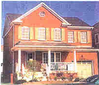
Example of a porch protrusion combined with a second storey build-over. The front porch and main building wall are the dominant visual features
